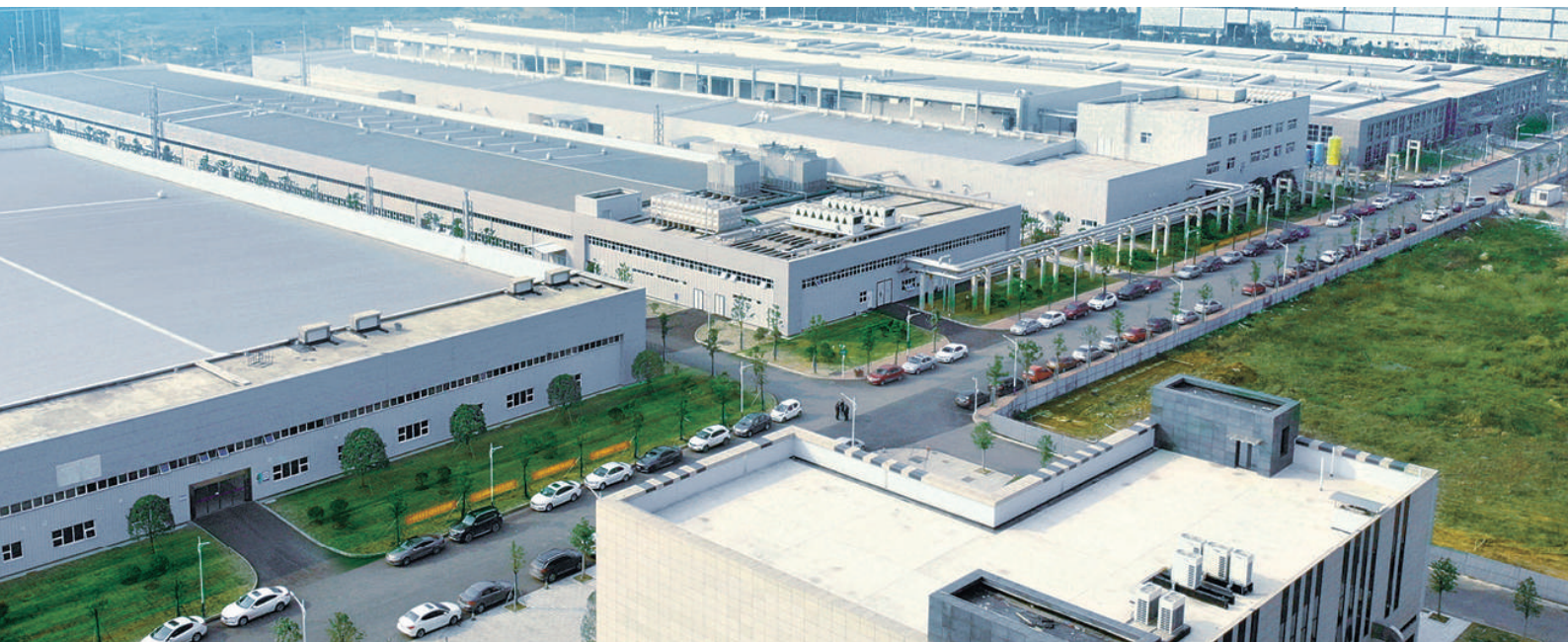
New ZCC Cutting Tools Industrial Park, Zhuzhou, China
